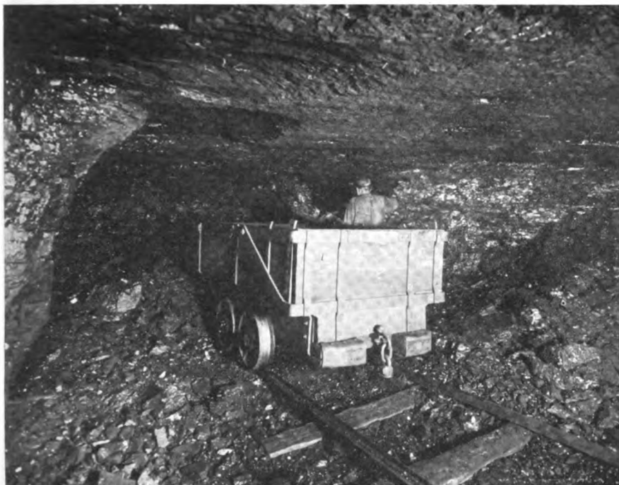
Miner loading at the face after coal has been shot down
