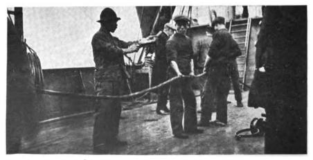
Splicing a broken cable before " paying " overboard  $${\tt Digitized}$ by $Google$$
