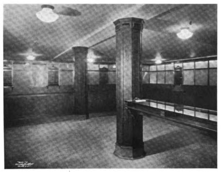
A corner of the banking floor The Mechanics & Metals National Bank, New York, showing collections, telegraph, cable and redemption department windows. The octagonal column in the foreground in this illustration is a dummy having nozzles or air outlets on the upper surfaces
