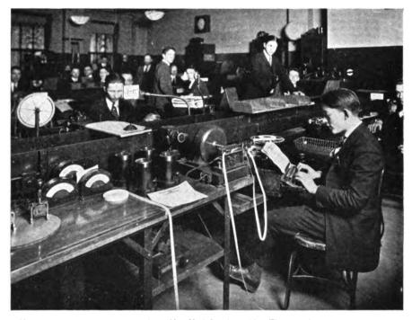
Here a message is being sent on a direct New York-London cable. The special typewriter perforates the tape, and transmission is effected by this tape passing through an automatic transmitter
