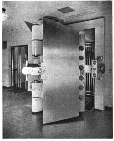
Rectangular vault door 36 inches thick, built by York Safe & Lock Co. for new Bowery Savings Bank vault
