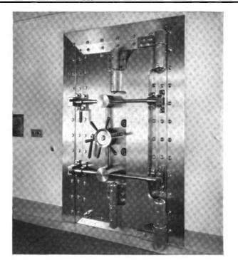
Main entrance to safe deposit and security vault Fidelity & International Trust Co., William & John Sts., New York showing YORK door in closed position with heavy polished steel hinge, pressure system, etc.
