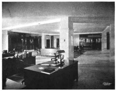
A section of the officers' quarters, Seaboard National Bank, New York, showing distributing air ducts which are at the ceiling between the interior columns and which have the appearance of ceiling beams. The noszles or air outlets are on the side of the ducts
