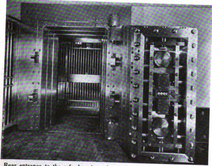
Rear entrance to the safe deposit vault of the Mechanics and Metals Bank -20 inch rectangular YORK door.
