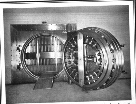
Standard 15 inch circular YORK door—entrance to safe deposit vault Bank of Manhattan, Jamaica Branch—security vault has rectangular door of same thickness.
