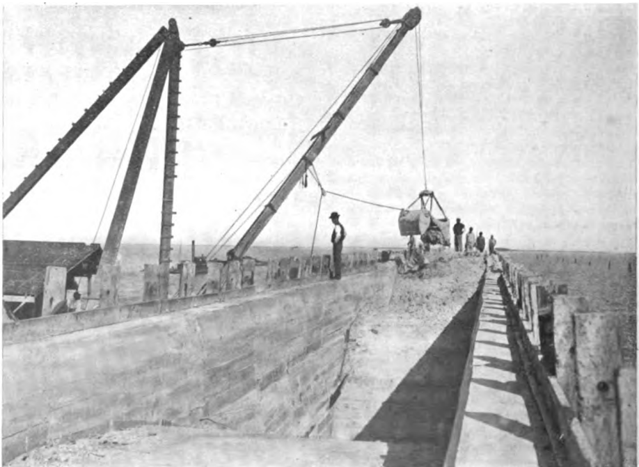
Long Key Viaduct.—Filling the last arch.
